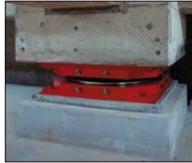
Figure1.2: Friction Pendulum Systems
